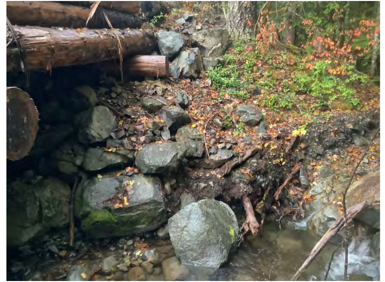
Right Bank Abutment when facing downstream
