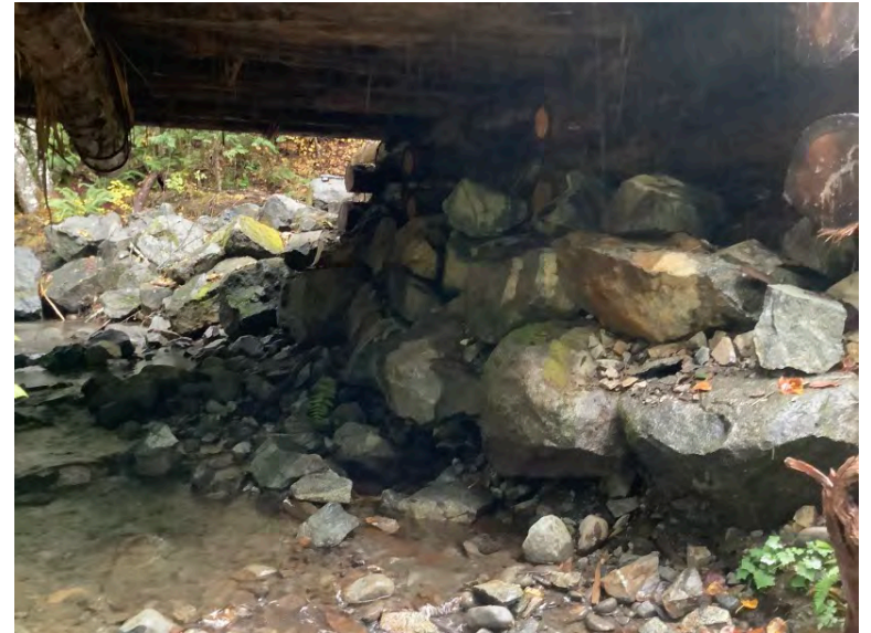
Left Bank Abutment when facing downstream
