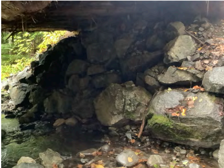
Right Bank Abutment when facing downstream
