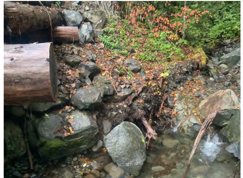
Right Bank Abutment when facing downstream
